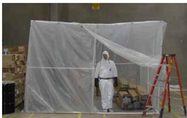
Photograph 2.2: EPSI Phoenix Facility - Containment Structure
