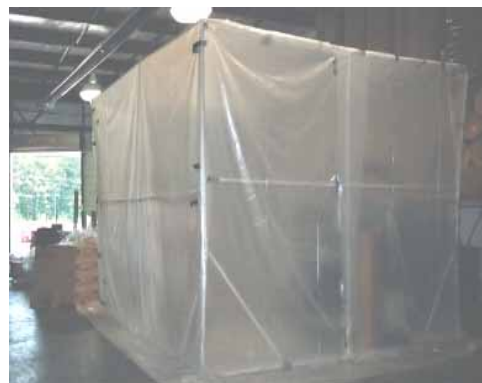
Photograph 2.4: AERC Ashland Facility - Containment Structure - Second Visit
