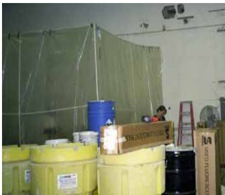
Photograph 2.3: AERC Melbourne Facility - Containment Structure
